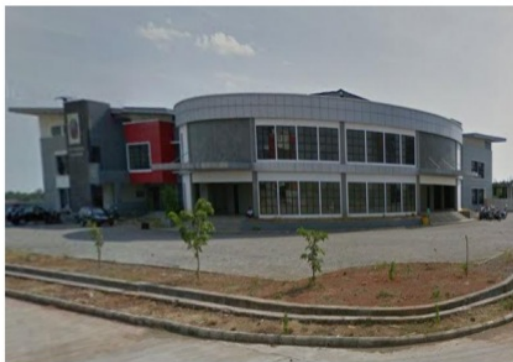
Fig.2. Electrical department building from left side
