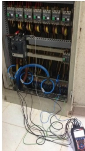
Fig.5. Installation of combined power measurement
